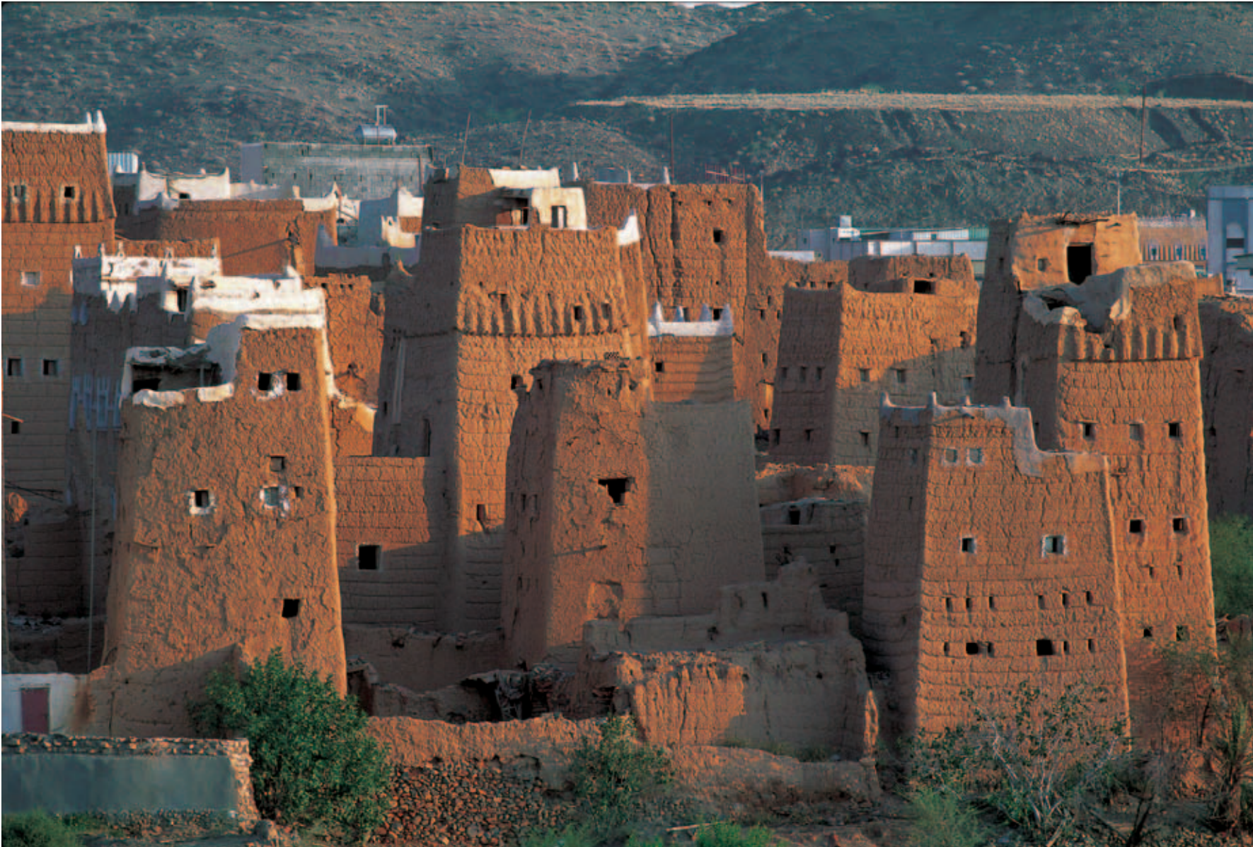
A house in Dhahran al-Janub, an oasis in the mountainous Asir province. Built by piling up rammed earth, its structure would have provided good protection in times of battle in the past.
